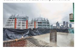
That is why more than 150km of REHAU's Thermally Activated Building Structure (TABS) system was installed to provide low energy passive cooling.
