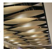
supporting structure, 4 metres above the mall floor. The custom support structure, comprising horizontal support rails and vertical suspension rods, was devised to
